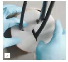
Before applying KÖSTER KB-Flex 200, a backing is installed in the penetration at a depth corresponding to the installation depth (consult Technical Data Sheet) using e.g. a common PU foam.
