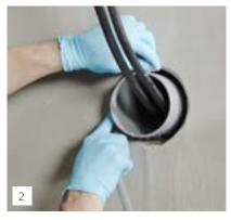
Next, insert a backing rod into the penetration, ensuring it reaches a depth that corresponds to the installation depth given in the Technical Data Sheet. Maintain a depth to width ratio of at least 1.5:1, with a minimum depth of 8 cm.
