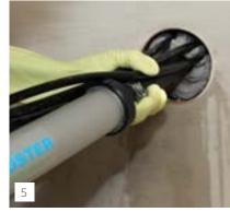
The KÖSTER KB-Flex 200 material is pressed into the penetration from back to front. Waterproofing made of KÖSTER KB-Flex 200 must be dimensioned so that the ratio of the depth (d) to the width (w) of the installed material is not below 1.5:1. The minimum depth should not be below 8 cm. The maximum diameter of the waterproofing is 300 mm.
