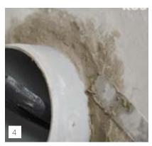
Finally, cover the exposed material with KÖSTER KB-Fix 5 to complete the sealing process.
