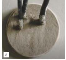
As an additional safeguard and to hold the pipe/cable centered, the exposed material is covered with KÖSTER KB-Fix 5.
