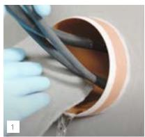
The application area flanks must be thoroughly cleaned with an abrasive pad and with KÖSTER Cleaning Brush from the inside so that they are free of dust, sand and other loose particles.
