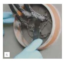
When sealing cable penetrations, jiggle the cables to reveal voids and re-press KÖSTER KB-Flex 200 into any eventual voids created. Ensure that the cable is tension free after finishing the sealing.
