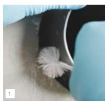
Begin by thoroughly cleaning the area between the structure and the pipe penetration using a KÖSTER Cleaning Brush or an abrasive scrubbing pad.
