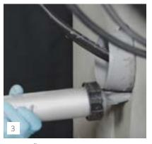
Apply KÖSTER KB-Flex 200 using a KÖSTER Special Caulking Gun equipped with a nozzle suitable for narrow spaces. Ensure the material is pressed evenly into the gap, either manually or with a KÖSTER Spatula.
