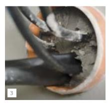
Finally, the penetration is resealed by pressing additional KÖSTER KB-Flex 200 around the cables.
