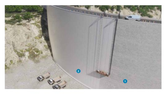
1 Substrate 2 Waterproofing layer TPO Aqua 2.5 Geo
